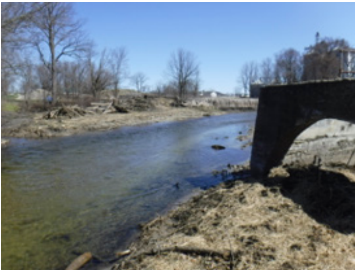
This picture was taken shortly after the dam was removed. Note the nice gravel bottom.
